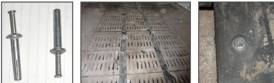
Figure 72 Use of stainless steel rivets and long metal plates to fill the fertilizer “holes” on the gestation slats
