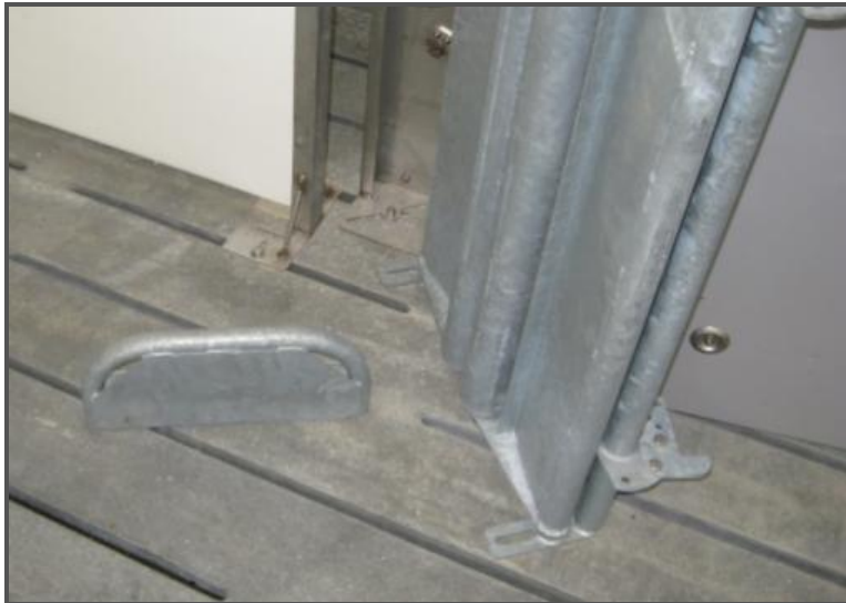
Figure 51 Clamp preventing lying down installed on floor in front of ESF exit gate
